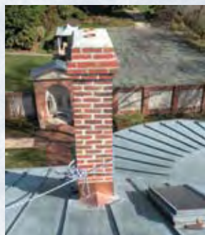
A historic Dumbarton House chimney is restored to eliminate water infiltration.
